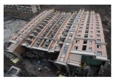
On June 27, 2009, Block 7, one of eleven 13-story apartment buildings... in Shanghai, toppled over, completely intact. The high-rise was still under construction, and luckily, most of the workers were able to evacuate the building when they felt it start to fall over. Unfortunately, one man wasted too many precious seconds collecting his tools. He was then forced to jump out of a window as the building began to go down. He fell to his death.
